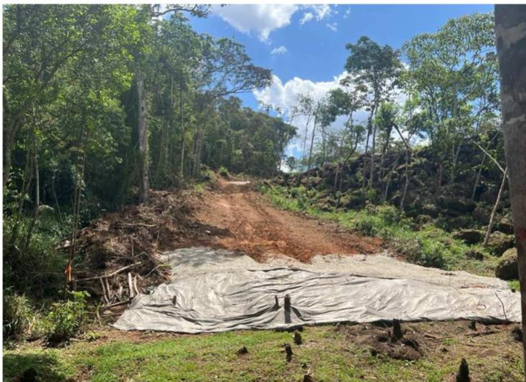
Photo 3: Xingú MI002 drill rig access (October 24, 2023)
