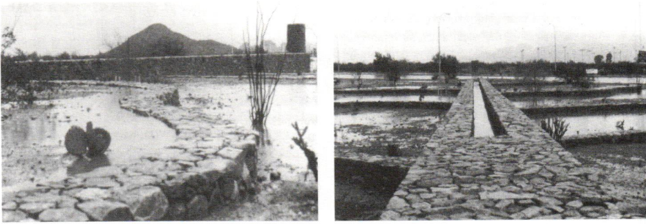
Papago Park City Boundary Project with rock terraces forming several water-harvesting pools, Phoenix, Arizona; Jody Pinto and Steve Martino, 1992. (From The Once and Future Park .)
