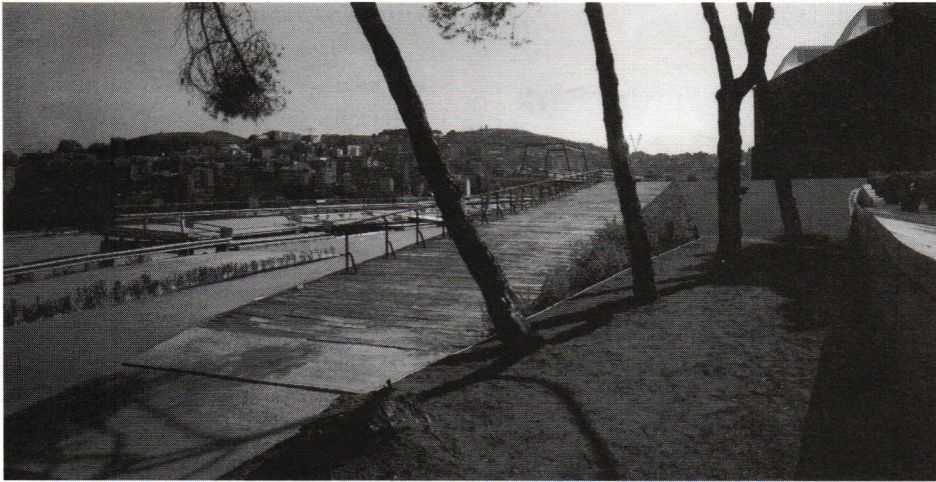
Vall d'Hebron, Barcelona; Eduard Bru, 1992. (From Quaderns de Arquitectura .)
