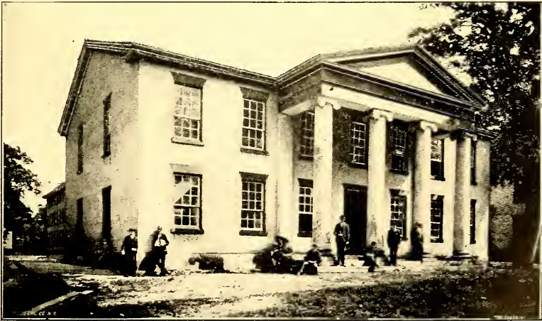
GERRARD HALL, SOUTH SIDE, BEFORE REMOVAL OF PORCH.
