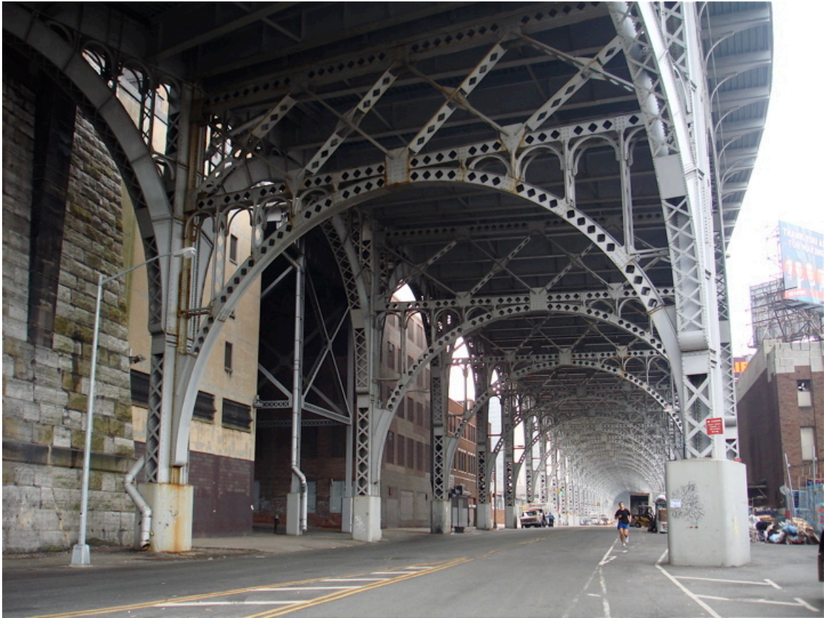
Figure 31 Under the viaduct in Harlem
