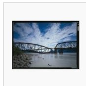
Collapsed " Million Dollar Bridge ", Alaska
