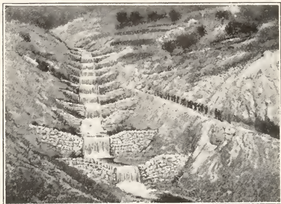
Working to prevent erosion after the removal of the forest in the French Alps.
