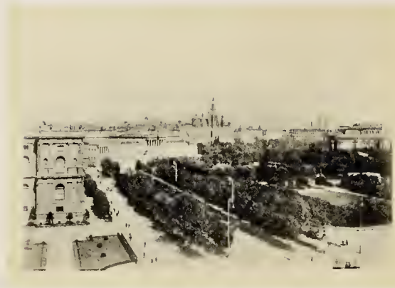
CXXXV. VIENNA. THE RINGSTRASSE, SHOWING THE PUBLIC BUILDINGS GROUPED ABOUT SQUARES AND GARDENS ALONG ITS COURSE.
