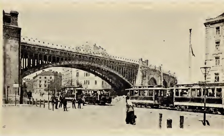
LXXVII. VIENNA. A RAILWAY VIADUCT PASSING OVER AN IMPORTANT STREET.
