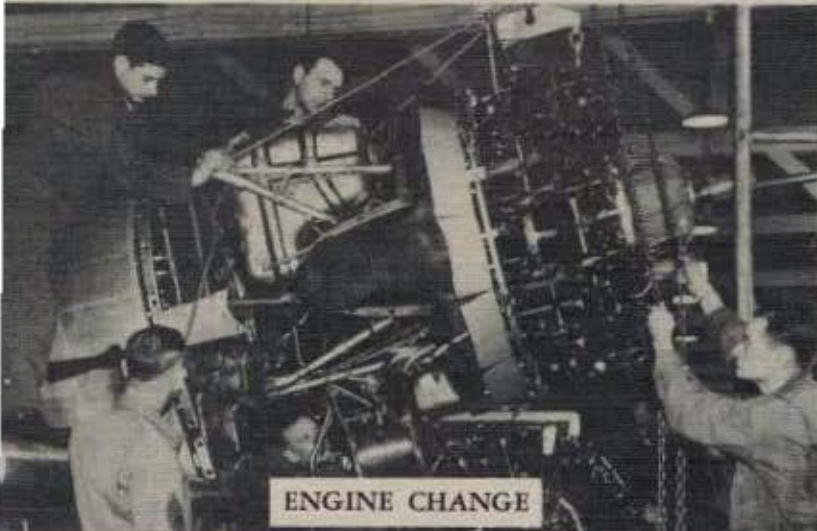
INSTALLING ENGINE
