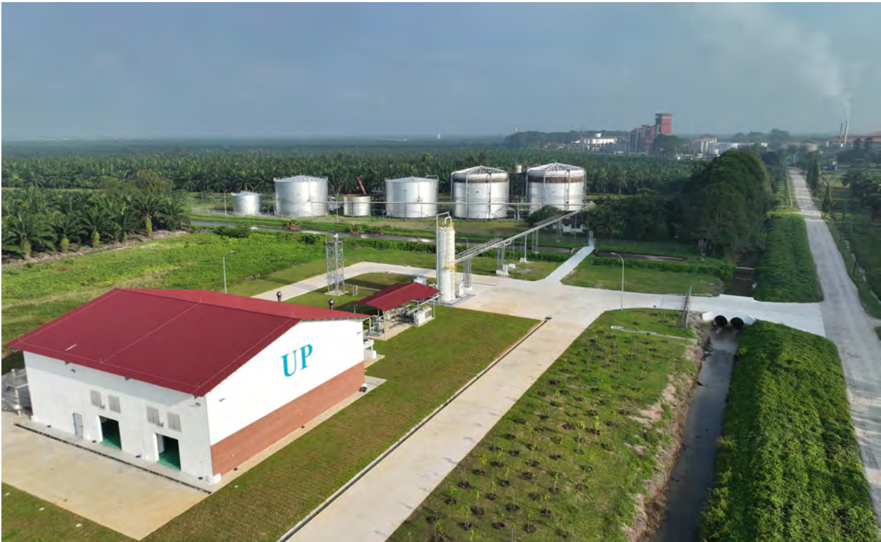
The newly commissioned Green Electricity Plant, further displacing the use of fossil fuels.
