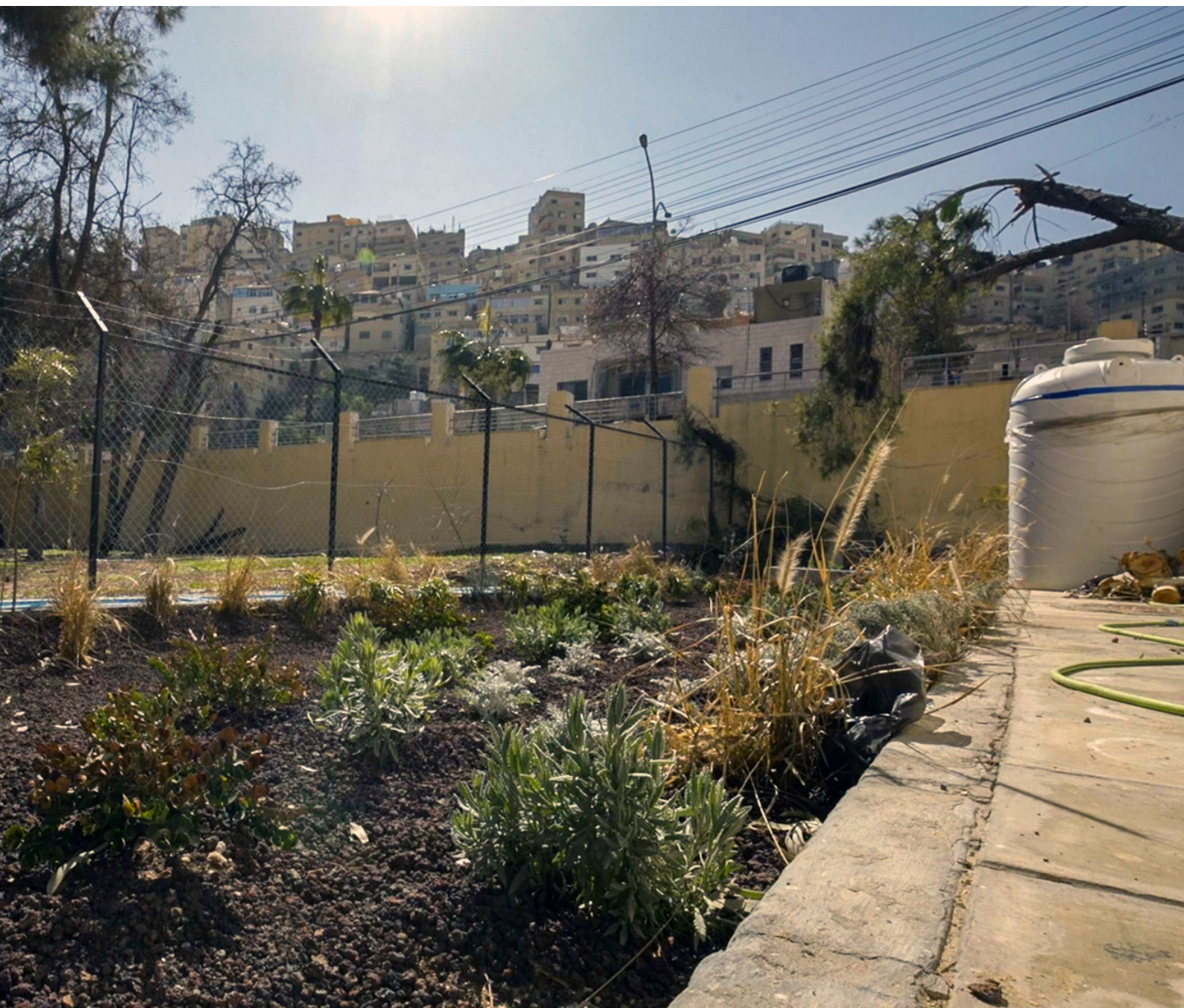
Figure 34. Rain Garden to Mitigate Flash Flood Risk in Affordable Housing Unit in Amman (Source: UN-Habitat, 2022)
