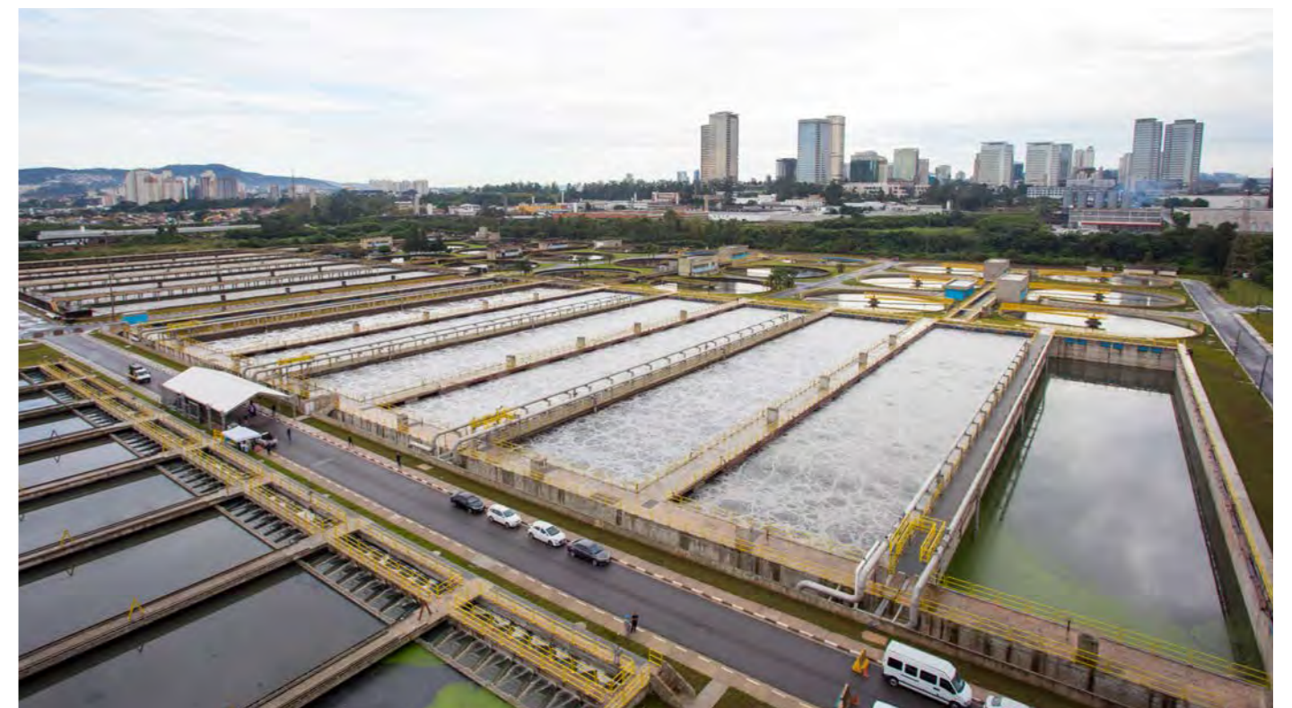
Piqueri Sewage Pumping Station.
