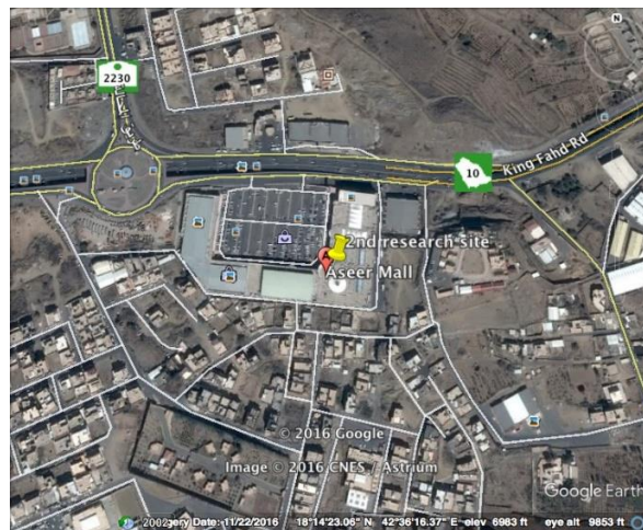
Figure 3-3. Aerial photograph of Asir Mall 2016 (Google Earth, 2016). Source: Google. (n.d).[Saudi Arabia, Asir Mall location]. Retrieved October, 2016, from https://earth.app.goo.gl/5Chw7
