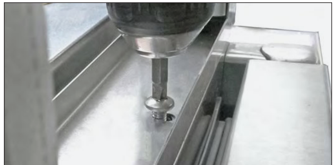
FIG. 10. Remove the screws from the metal channel.
