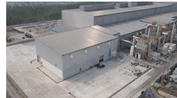
Side well furnace building
