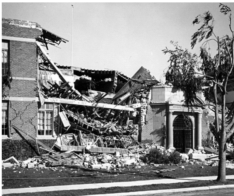
Figure 1 Jefferson Junior High School damage after the 6.4 magnitude 1933 Long Beach earthquake.
