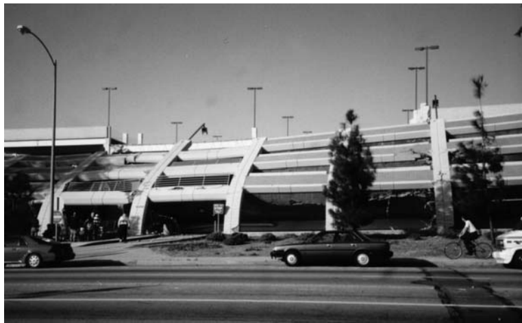
Figure 3 California State University Northridge parking structure built in the early 1990s collapsed after the 6.7 magnitude 1994 Northridge earthquake.
