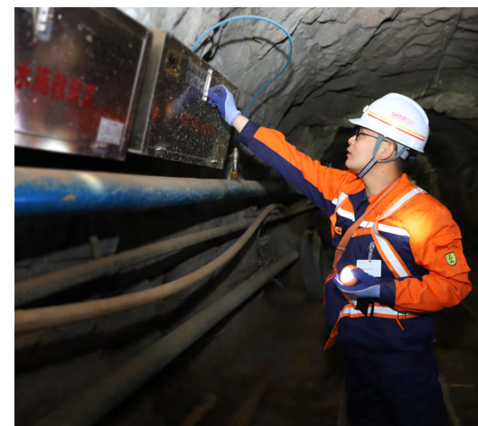
Check the water supply facilities
