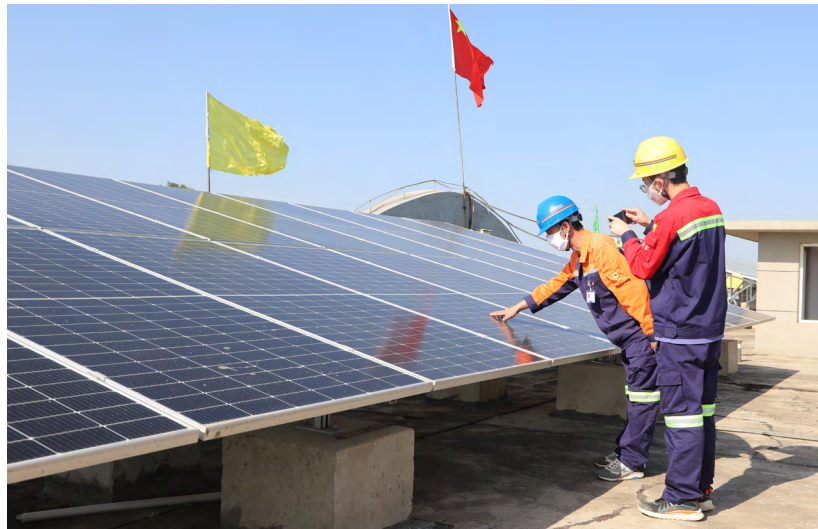
Henan Found installing photovoltaic power generation facilities
