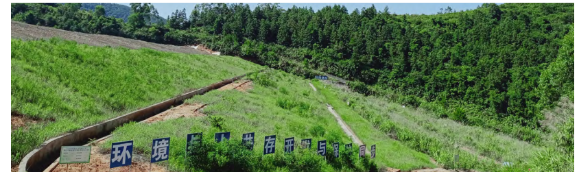
TMF dam slope after reclamation
