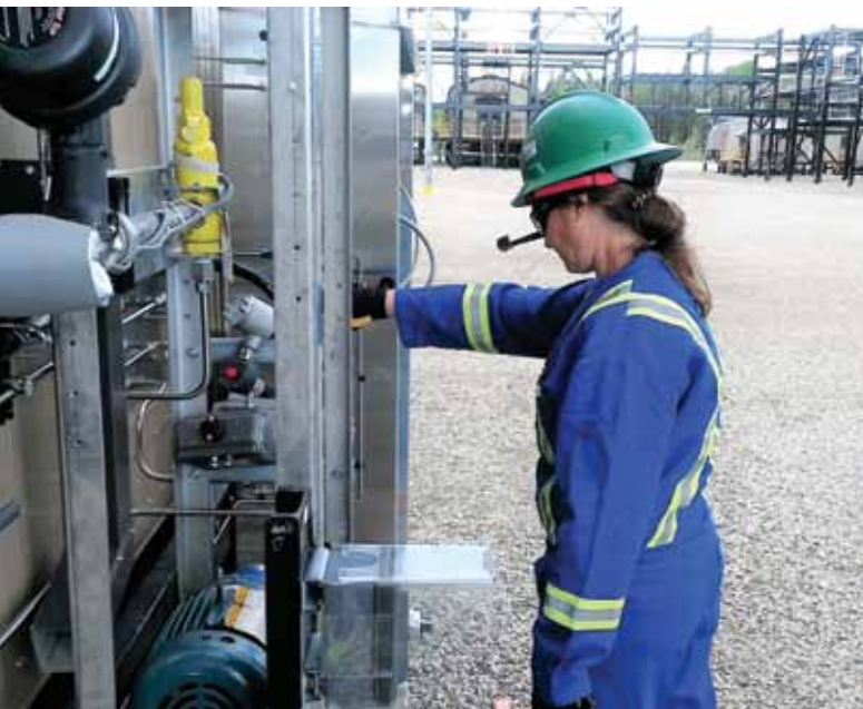
A field engineer wearing an AR headset inspects critical equipment at a chemical plant with the help of an engineering team watching a livestream video and providing remote support.
