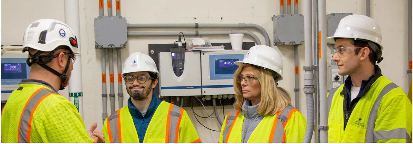
Visitors get a look at investments in Pennsylvania American Water's Coatesville facility.
