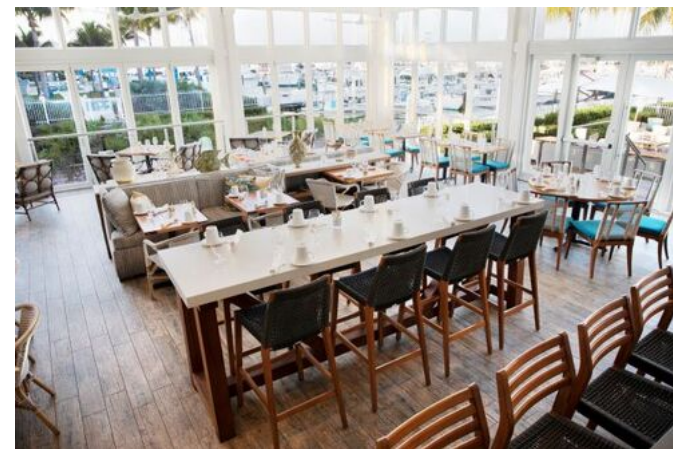
Hurricane-force storm windows installed at the Oceans Edge Resort and Marina (Key West, FL).
