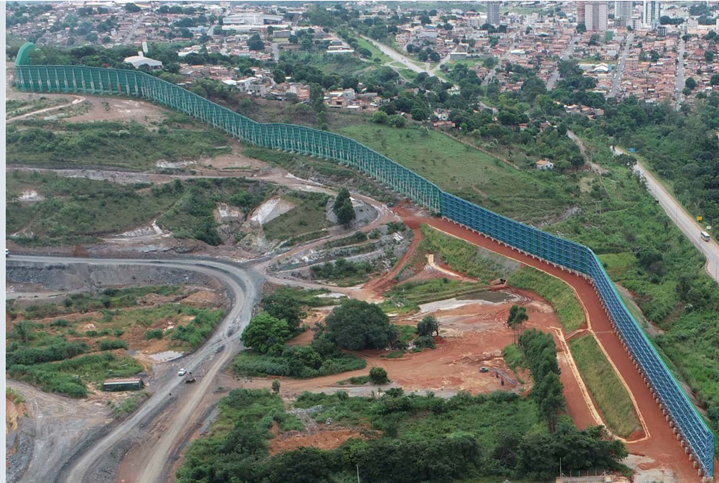
Aerial image of the acoustic barrier in Paracatu
