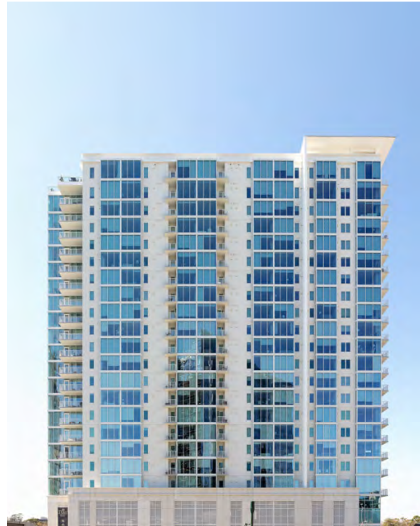
MAA Lenox | Atlanta, GA | NGBS-certified MAA Lenox received consecutive ENERGY STAR certifications in 2021 and 2022.
