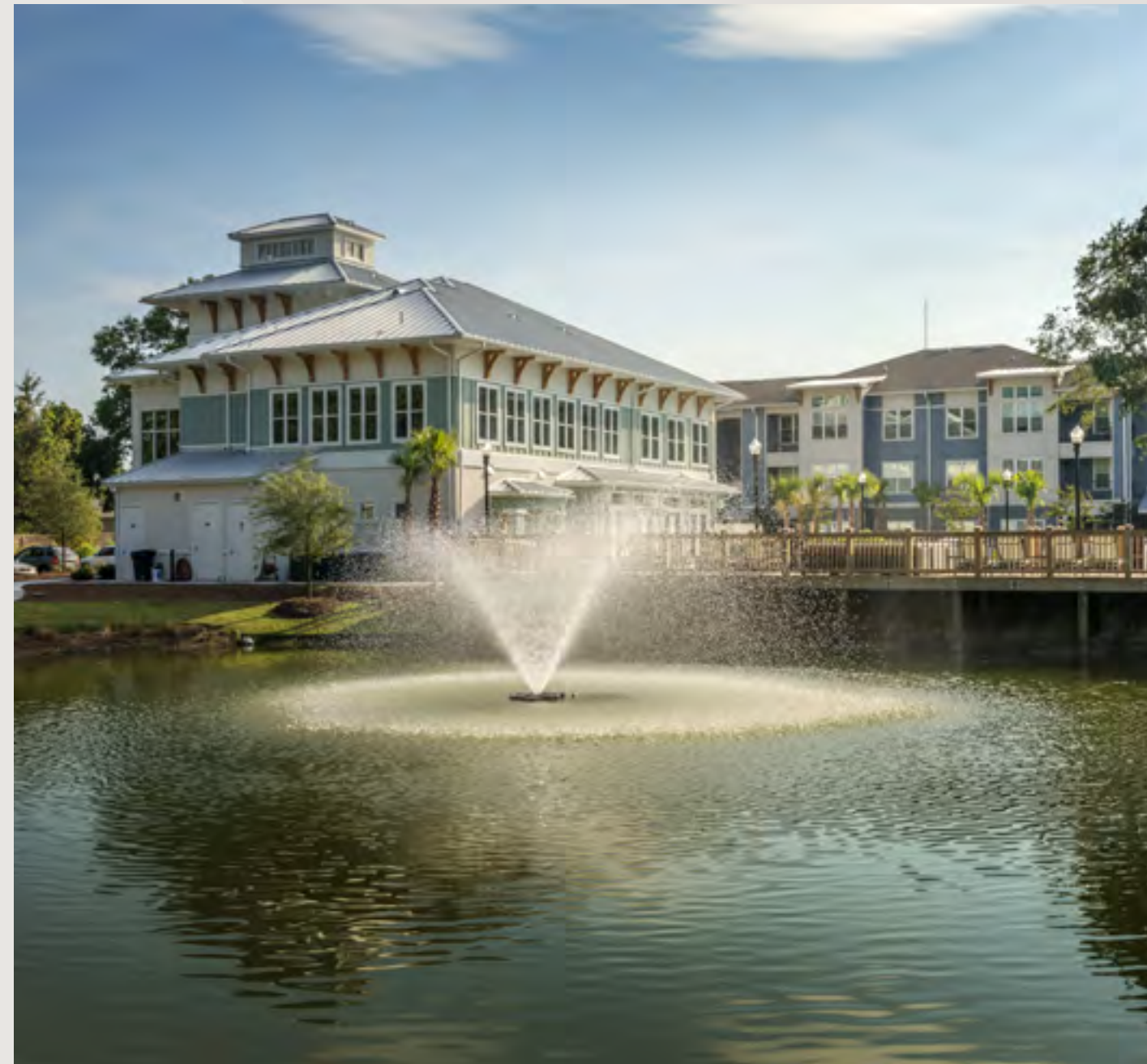
MAA Rivers Walk | Charleston, SC | Through our use of an on-site retention pond for irrigation at MAA Rivers Walk we have significantly reduced our overall potable water usage resulting in cost savings for the community.
