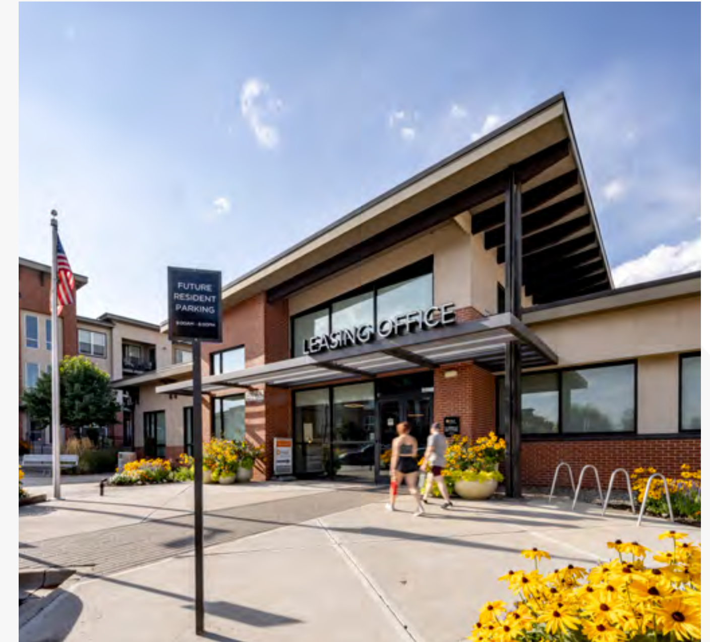
MAA Westglenn | Denver, CO | Residents of our NGBS-certified MAA Westglenn community have access to the many features that support healthy lifestyles and resource efficiency.
