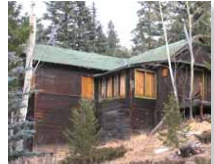
Wigwam Tea Room before restoration
