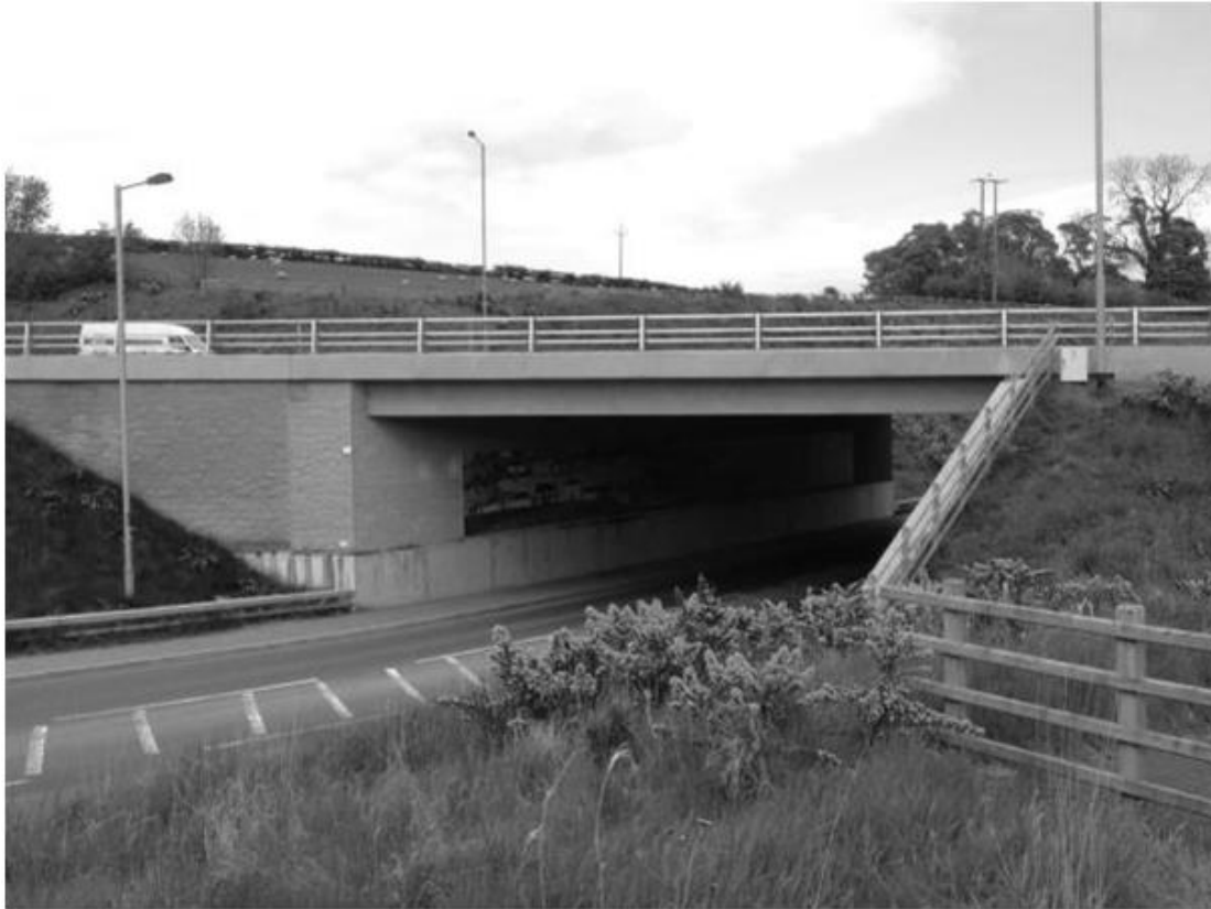
Figure 11 Loughbrickland Test Bridge
