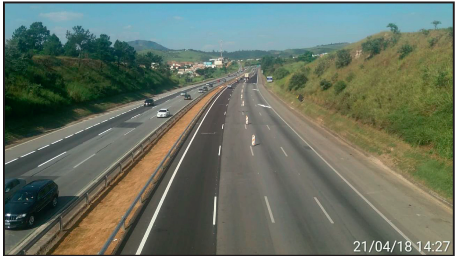
FIGURE 8: Additional lane to the left opened to traffic.
