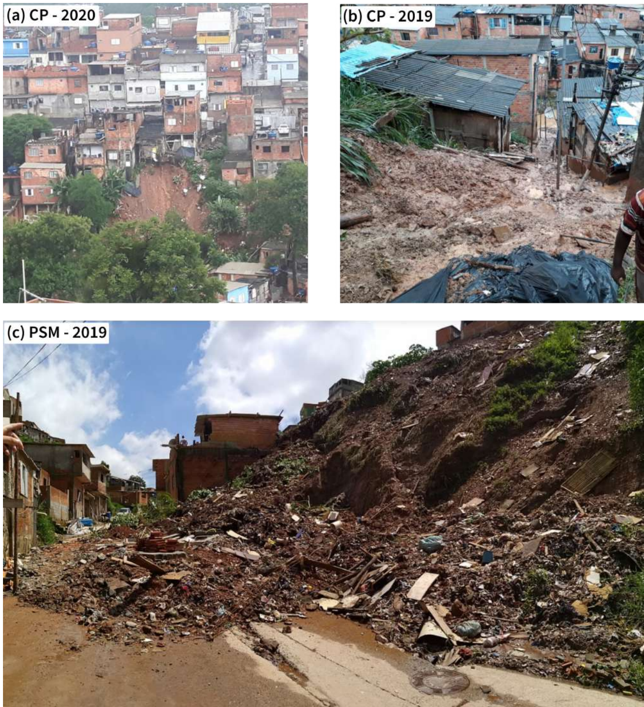
Figure 12. Occurrences of small landslides in the study areas. (a) East slope of CP area in February 2020. (b) Southwest slope of the CP area in February 2019. (c) East slope of PSM area in February 2019. The yellow dot on the insets shows the landslide location.
