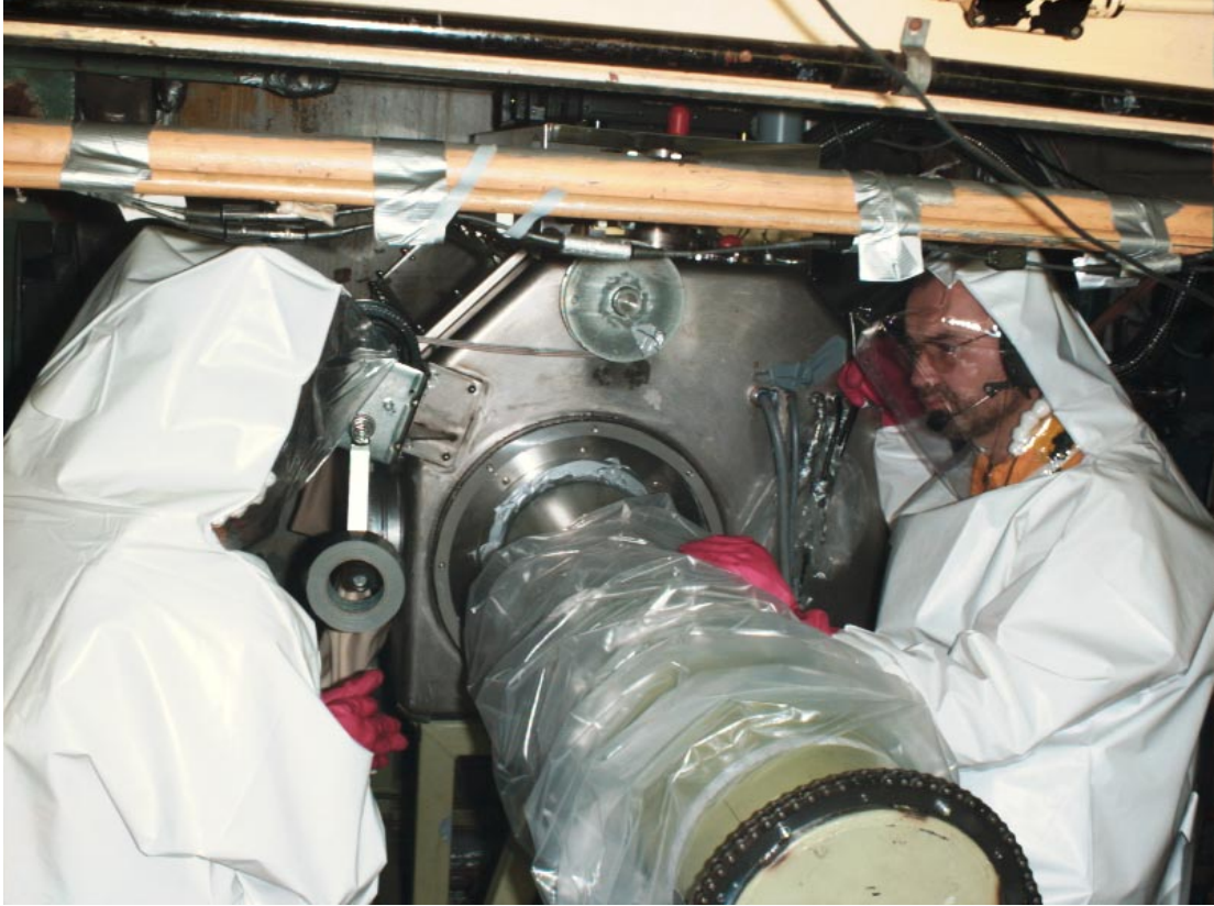
Fig. 4. Drilling site installation and locking out of a sample
