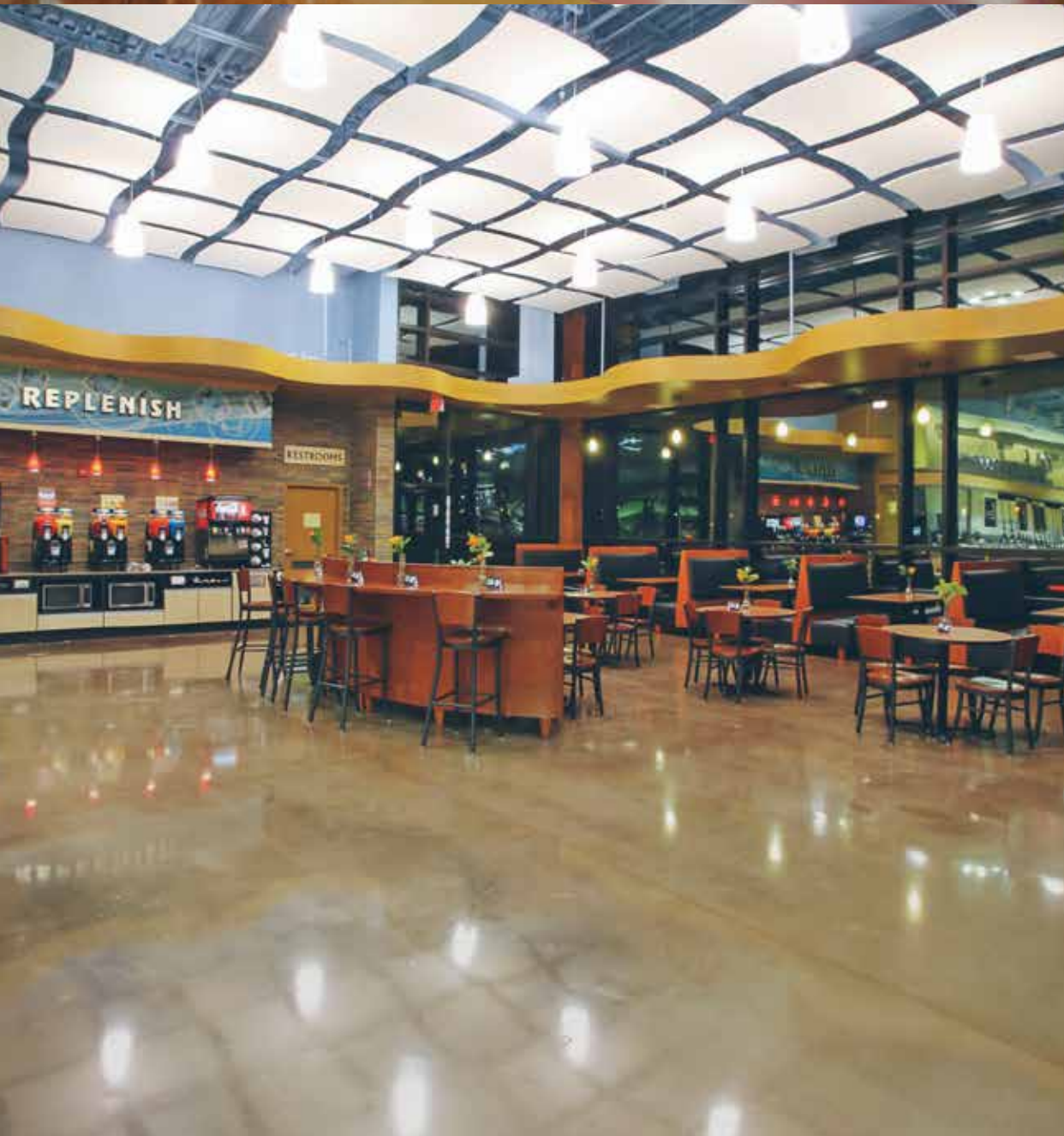
Price Cutter // Springfield, MO colored with GemTone Stain Light Roast // densified with LS // protected with LSGuard
