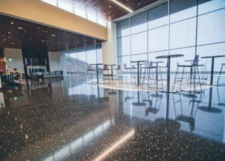
Skyline College Environmental Science Building // San Bruno, CA colored with Integral Color for Overlays in Black // densified with LS // protected with LSGuard
