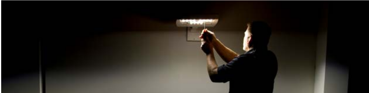
Energy-efficient lighting installation
