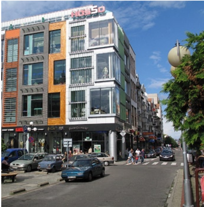
Glass facade instead of iron curtain: the modern Kolobrzek
