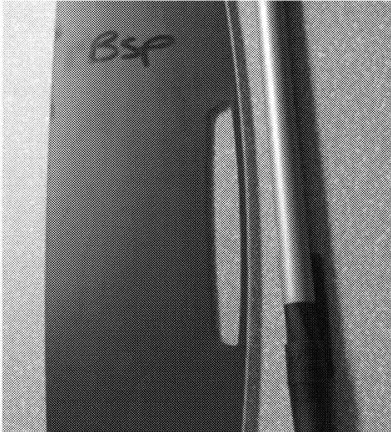
protect exposed edges by applying a film on window to protect exposed silver
