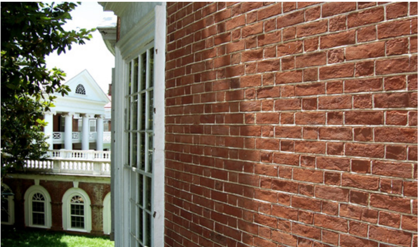
EAST ROTUNDA COURTYARD
