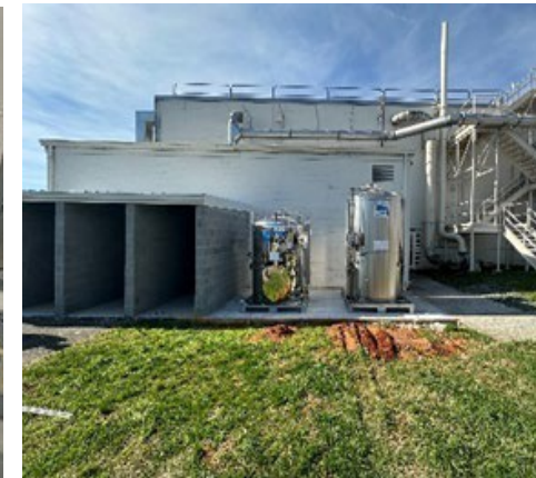
Supply Gas Installed
