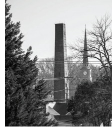
The Metrolina Warehouse | Carolina Asbestos factory in Davidson. Credit: David Boraks | WFAE
