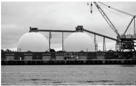
Two large domes at the Port of Wilmington store wood pellets manufactured in North Carolina before they are shipped to Europe to be burned as energy. Credit: David Boraks | WFAE
