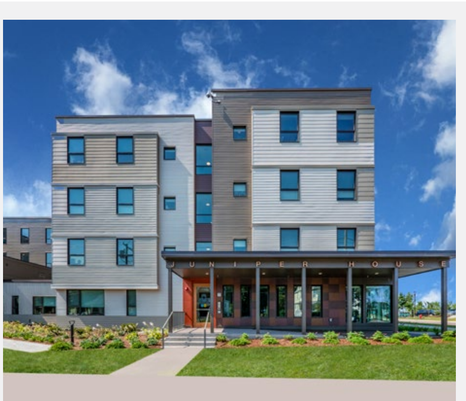
Juniper House, Cathedral Square Corp Senior housing with 7 units targeted for homeless people Burlington, Vermont
