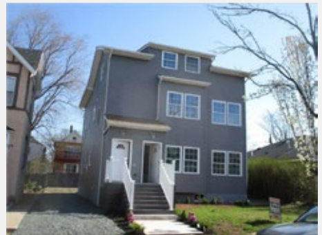
Powers Street Project, Triple C Housing Two three-bedroom units for families with special needs New Brunswick, New Jersey
