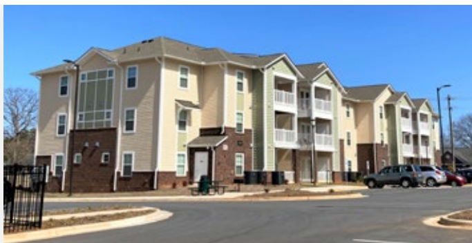
Muir's Landing, Affordable Housing Management Greensboro, North Carolina
