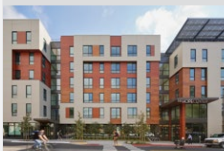
Hope Center, Berkeley Food & Housing Project (BFHP) with BRIDGE Housing
