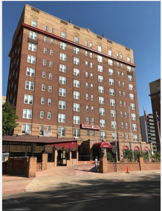
The Colburn, Gorman & Company LLC Conversion of SRO to efficiency units for homeless individuals Denver, Colorado
