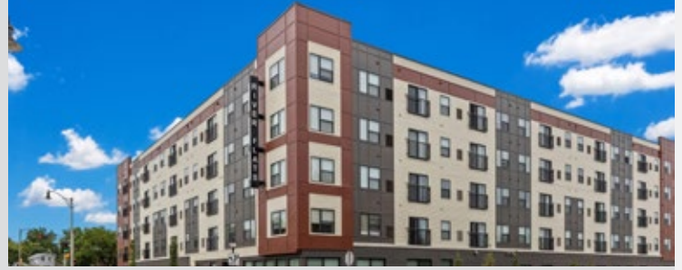
River Flats, The Commonwealth Companies 19 units of supportive housing Janesville, Wisconsin
