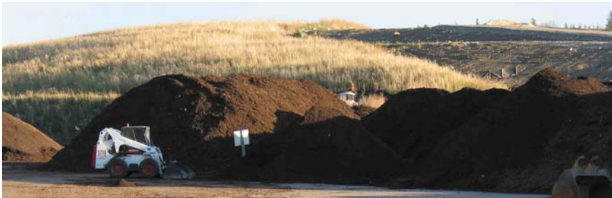
Figure 22. Compacted garbage is ready for a cover of soil. The dumped soil will be spread across the garbage to create a refuse cell. The soil-covered slope in the background is underlain by many refuse cells.
