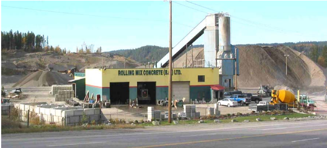
Figure 13. Concrete plant and sand-gravel quarry on Foothills Boulevard. Sand and gravel are quarried from the forested flat-topped bench (an ancient river plain) in the background.
