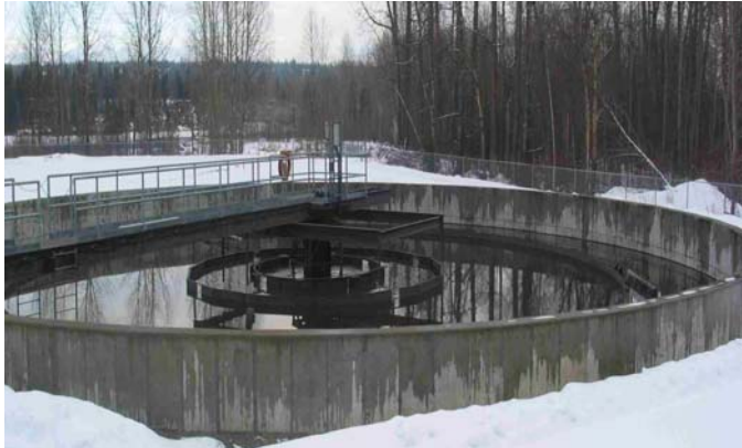
Figure 19. More solids settle out in large tanks (clarifiers).
