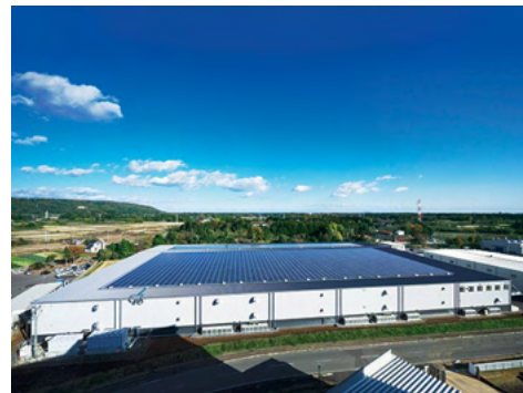
MJ Logipark Tsuchiura 1
