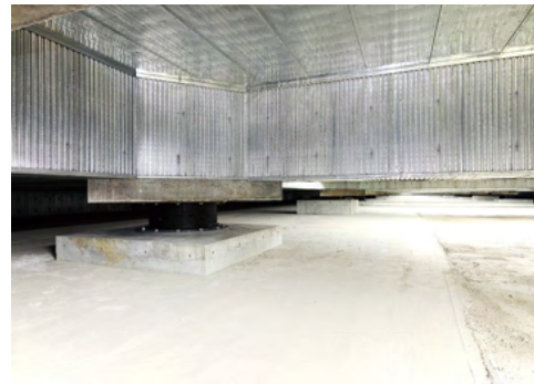
Seismic isolators
