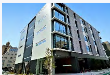
The new MEIDEN KOHSAN head office
