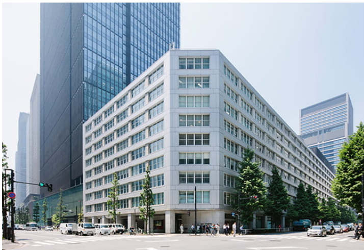
Otemachi Building before renovation
