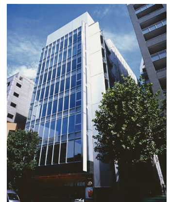
JRE Higashi-Gotanda 1-Chome Building
