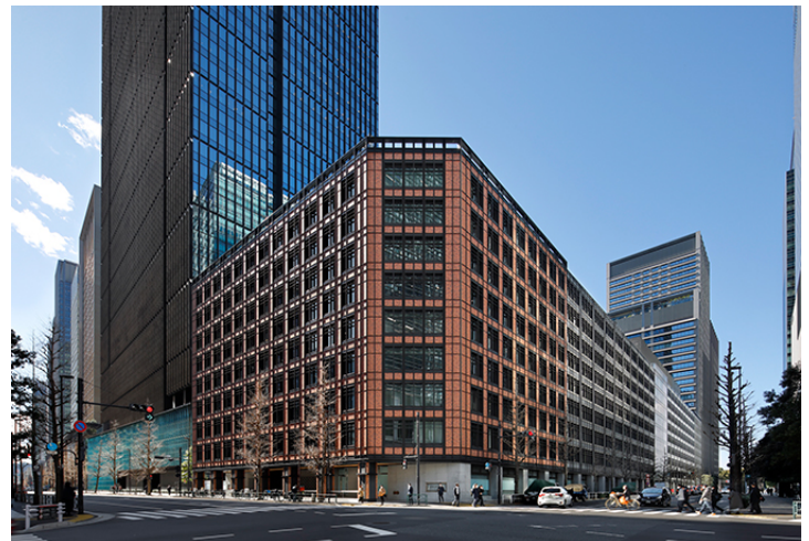
Otemachi Building after renovation
