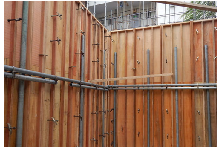
Example of formwork panels in use
