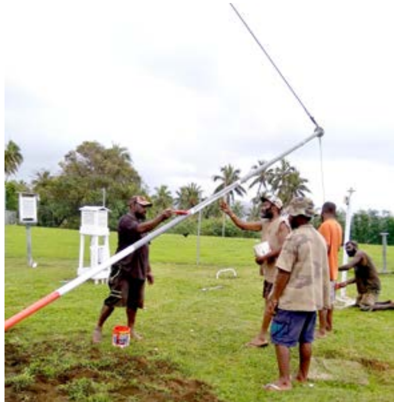
Installation of weather and climate monitoring systems in Vanuatu.
