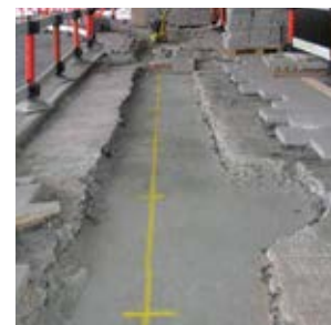
Shallow mount footings require minimal excavation and concrete.
