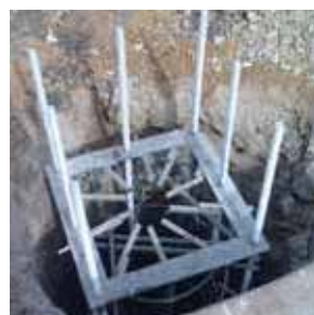
Concrete footings preparation for swing gates
