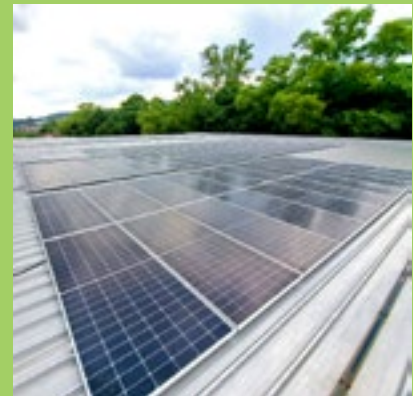
IBS Precast Concrete Factory @ Nilai
