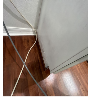
Lower Cabinets End Panels #1
