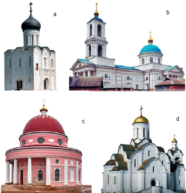
Figure 5. Examples of typical church constructions: a - chetverik, b - ship, c - rotunda, d - cross-in-square (from: www.iamruss.ru )
