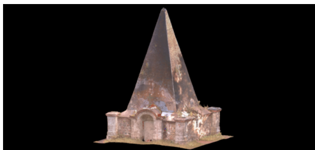
Figure 9. Point cloud of the building (created by M. Bura).
