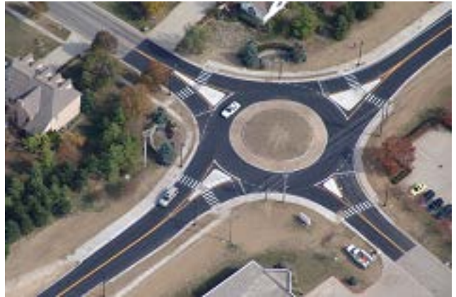
Figure 9-5: Roundabout at Lakota Drive West and Eagleridge Intersection in Butler County
