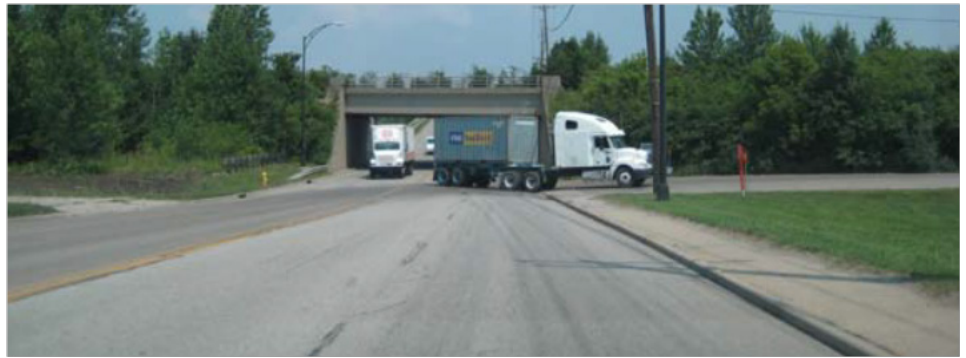
Figure 8-1: East Sharon Road Entrance to Norfolk Southern Railroad's Sharon Intermodal Yard
