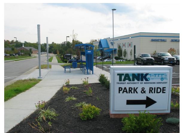
Figure 10-5: TANK Mt Zion Road Park & Ride
