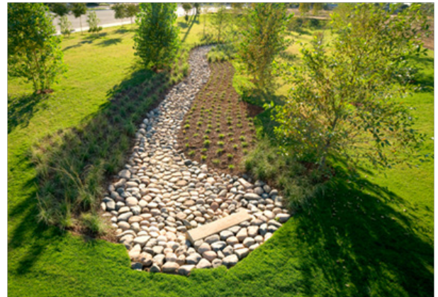
Figure 4-7: Example of a Bioswale Source: www.blog.lpainc.com
