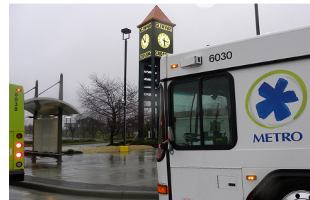
Figure 10-8: Glenway Crossing Transit Center
