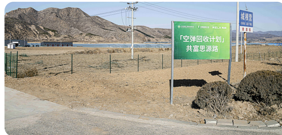
Recycled pods are used in the construction of rural roads
