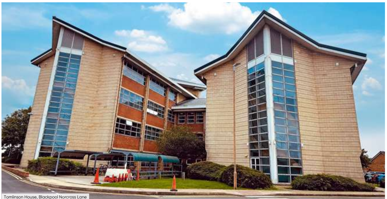
Tomlinson House, Blackpool Norcross Lane
