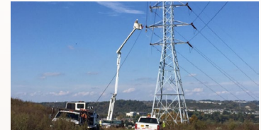
Figure A-38. Tower reconductoring.
