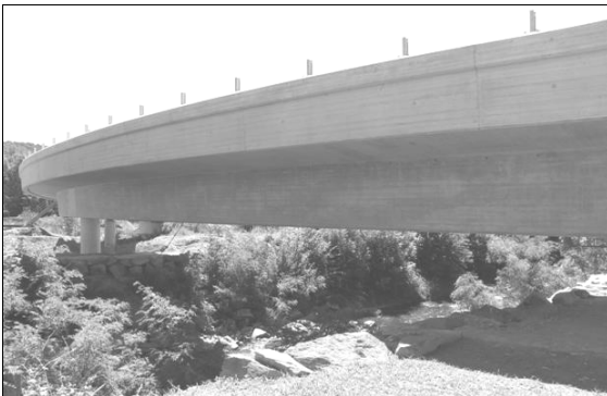
Figure 25: View of the main span of Ricciolo viaduct.
